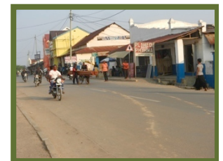
Newly paved roads in Kindu
